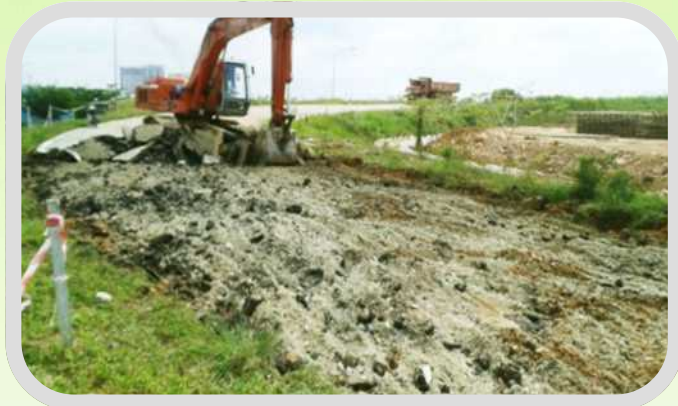
Stage 1 : Excavation works including removal of premix
