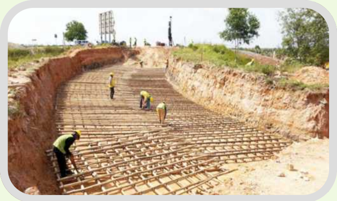
Stage 2 : Bamboo Installation Works
