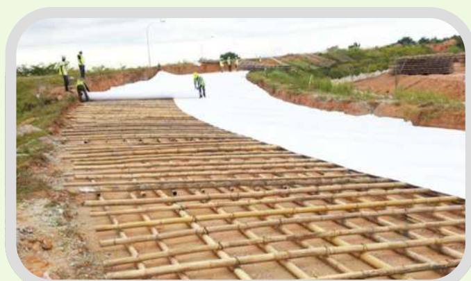
Stage 3 : Laying Geotextile
