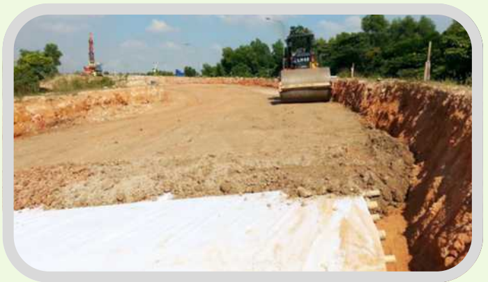
Stage 5 : Ground Compaction
