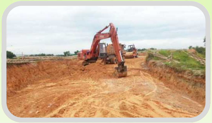
Stage 4 : Backfilling Works
